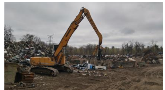
Two of the six Liebherr material handlers pick scrap at Moffatt’s busy yard in Campbellville, Ontario.
